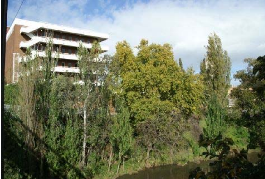
The current MFB building from the Yarra side. Imagine the new development - 5 stories higher - stretching across the whole width shown in this photo!
